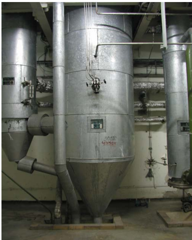
Evaporator for treatment of low - active \beta - \gamma liquid wastes
