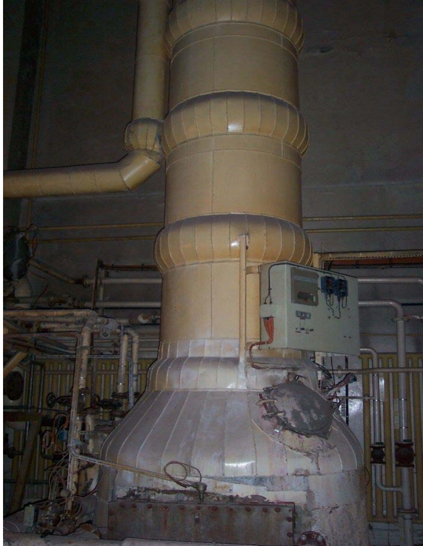
Evaporator of the STDR Magurele liquid waste treatment installation
